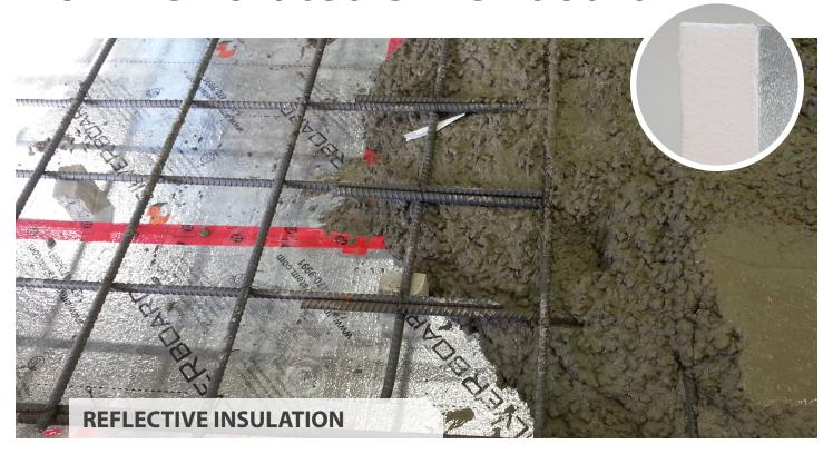
SilveRboard (SB) is a non-structural, rigid insulation board made from closed cell Expanded Polystyrene (EPS) with a layer of reflective metalized polypropylene film laminated on each side.
